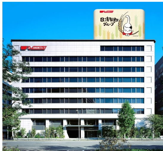
The office floors will be remodeled.
